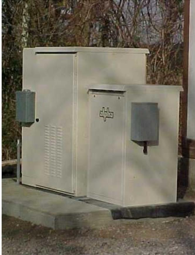
*Figure 4. Installed telecom genset collocated with RT. Genset is the smaller enclosure on the right of the figure.*
